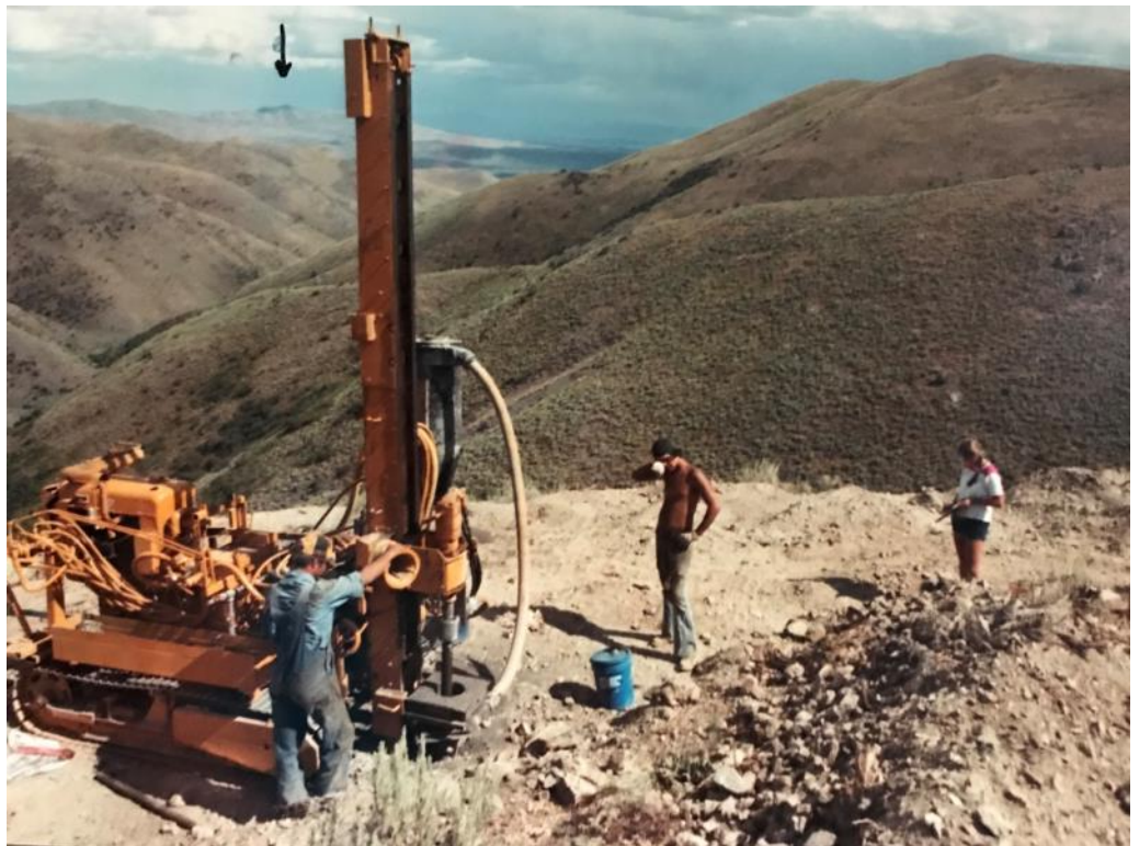
Drilling for barite, Beaver Peak, Elko County. Swales Mtn in background. Note the lack of PPE.
